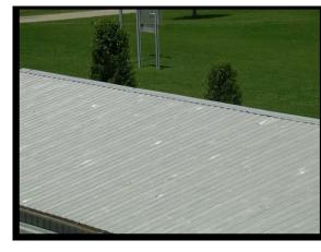
While not all hail dents to rooftop metals are harmful, inspecting these adjacent services can give credence to actual hailstone sizes and the severity of a questioned hail event.
