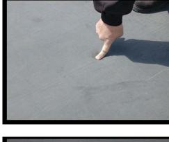
Non-reinforced EPDM has great flexibility properties, while underlying insulating substrates such as ISO-Board have low impact ratings. This combination can
