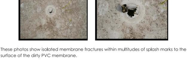
However, mere "splash-marks", in-and-of-themselves, on a roof system's surface does not necessarily indicate surface or membrane damages.
