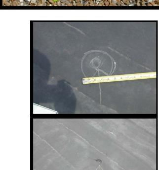
splash marks would be recommended to feel and inspect for membrane fractures
