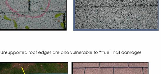
True hail impact damages will cause distinct impact compression marks which bruise the bitumen, fracture the reinforcing mats and cause significant and pronounced point
