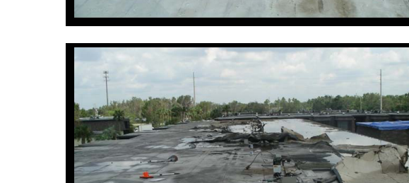
Catastrophic roof damages sustained by 90 mph straight-line winds in St. Louis Missouri in 2006.
