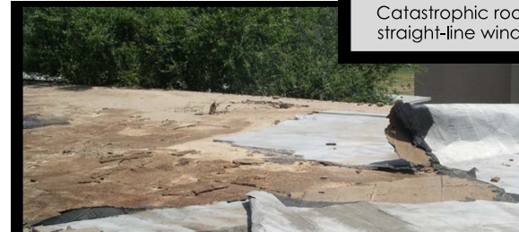
Catastrophic roof damages sustained by 100+ mph Hurricane Charley winds in Orlando Florida in 2003.
