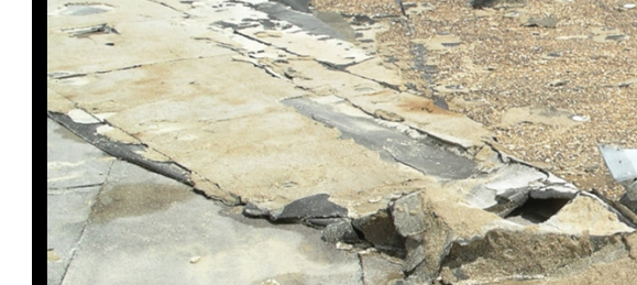
Catastrophic roof damages sustained by 90 mph straight-line winds in St. Louis Missouri in 2006.
