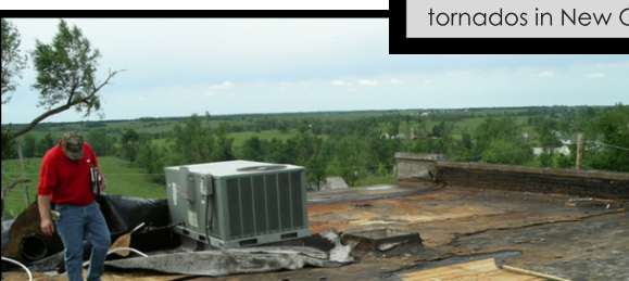
Catastrophic roof damages sustained by F-3 tornadoes in New Cambria Missouri in 2004.
