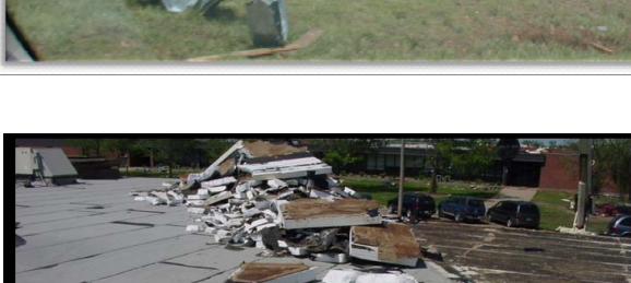
Catastrophic roof damages sustained by F-3 tornadoes in Carl Junction Missouri in 2003.
