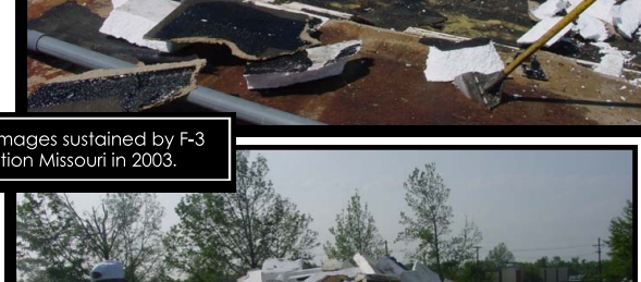
Catastrophic roof damages sustained by F-3 tornadoes in Carl Junction Missouri in 2003.
