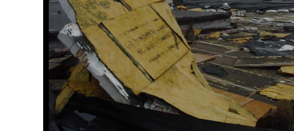
Catastrophic roof damages sustained by F-3 tornadoes in Carl Junction Missouri in 2003.
