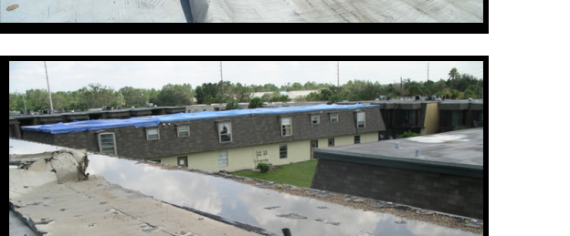
Catastrophic roof damages sustained by 90 mph straight-line winds in St. Louis Missouri in 2006.
