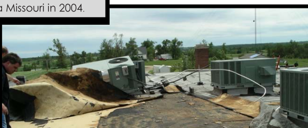
Catastrophic roof damages sustained by F-3 tornadoes in New Cambria Missouri in 2004.
