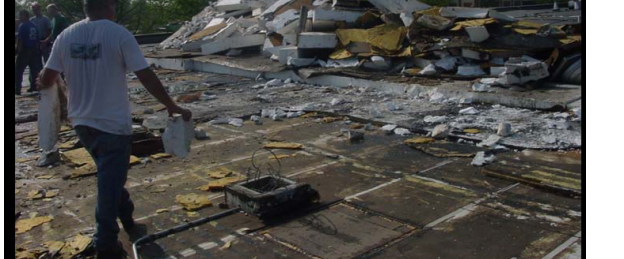
Catastrophic roof damages sustained by F-3 tornadoes in Carl Junction Missouri in 2003.
