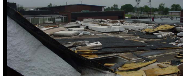
Catastrophic roof damages sustained by F-3 tornadoes in Carl Junction Missouri in 2003.
