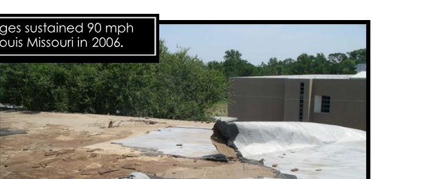
Catastrophic roof damages sustained by 90 mph straight-line winds in St. Louis Missouri in 2006.
