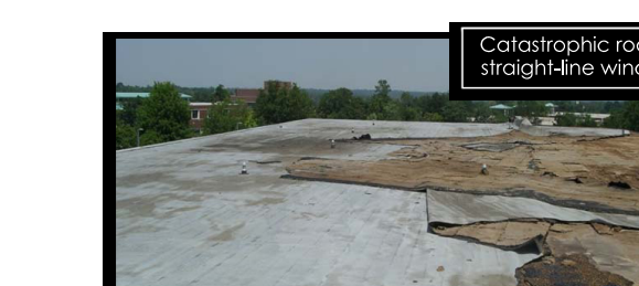
Catastrophic roof damages sustained by 90 mph straight-line winds in St. Louis Missouri in 2006.
