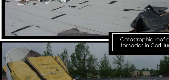
Catastrophic roof damages sustained by F-3 tornadoes in Carl Junction Missouri in 2003.
