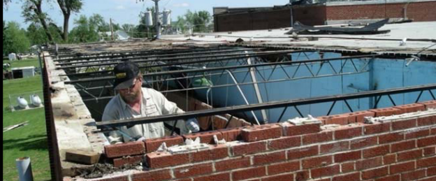
Catastrophic roof damages sustained by F-3 tornadoes in New Cambria Missouri in 2004.
